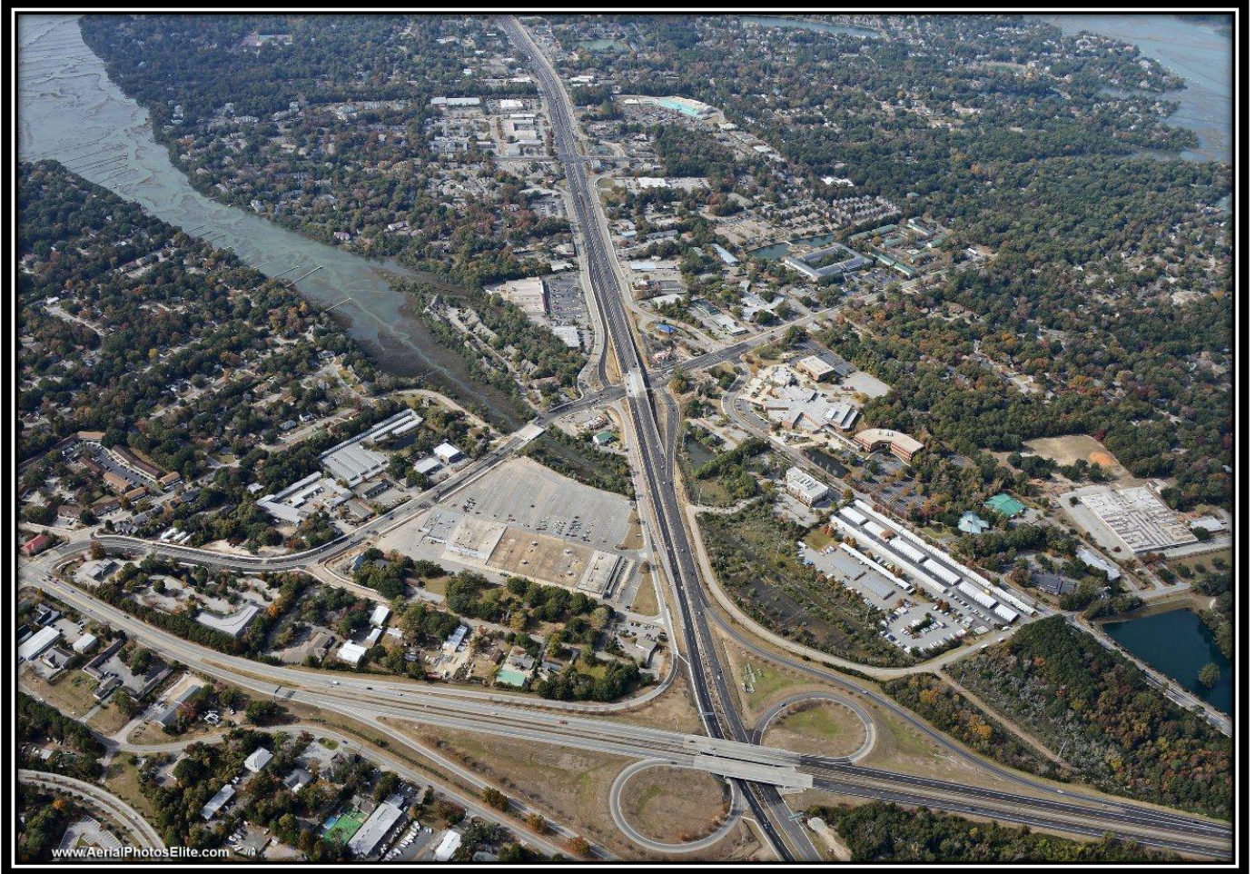
Improvements to Johnnie Dodds Boulevard.
